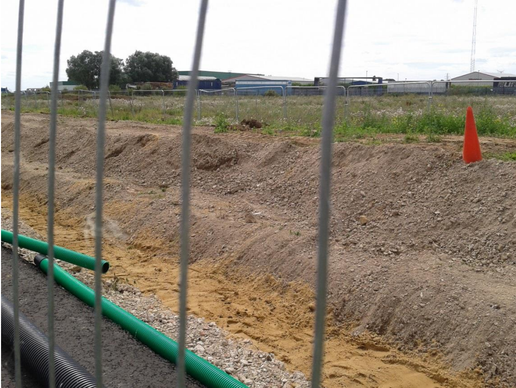
Plate 2: A culvert is currently being installed along the track in Boston 2
