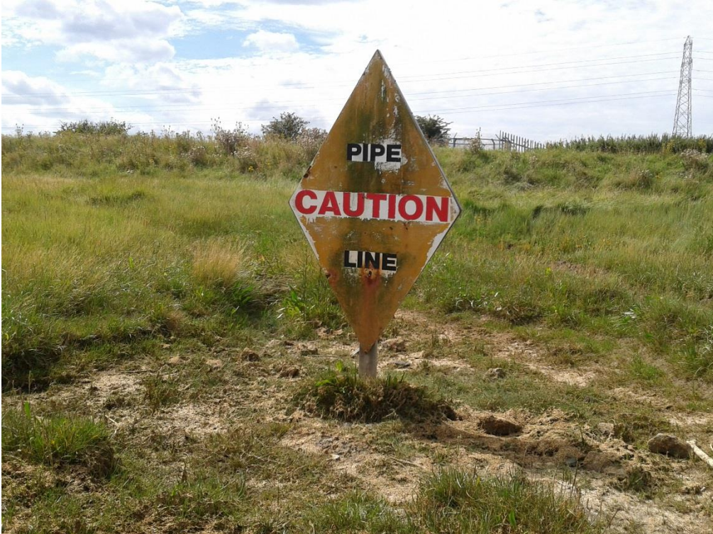
Plate 4: A sign marking location of a pipe line
